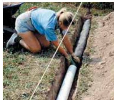
Figure 71: Underground Refrigerant Piping.
