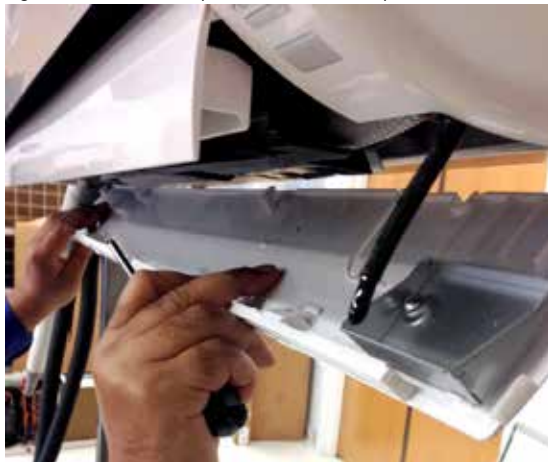
Figure 56: Removal (and Reattachment) of Bottom Panel
