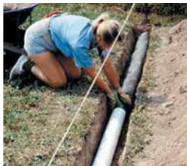
Figure 33: Underground Refrigerant Piping.
