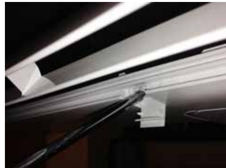
Figure 55: Remove Screws from Bottom Panel
