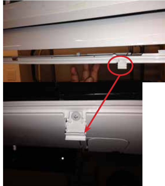
Figure 54: Latch over Screws on Bottom Panel, Indoor Unit
